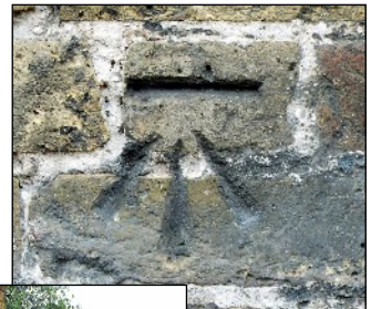
The cut benchmark on the side of the building at the corner of Victoria Road and Thanet Road
