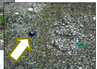
Close-up of rivet benchmark also showing an incised the arrow mark
