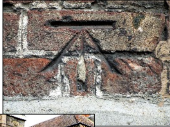
The cut benchmark on the side of the building at the corner of Addington Street and Hawley Square
